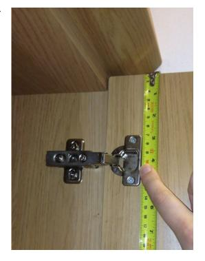
Then measure from the bottom edge of the door to the centre of the bottom hinge hole for the bottom hinge position. It is important to measure every door as some hinge hole positions may vary.
