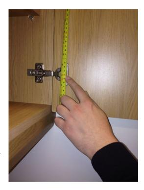
The hinge holes are drilled as a standard 35mm diameter hole. You don't need to worry about the measurements in from the side edge of the doors as this measurement is always standard at 22.5mm to centre of hole.
