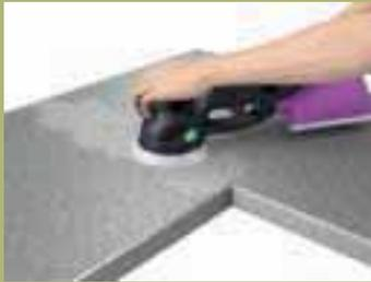
Ensure the sander is moved constantly during sanding operations. Holding the sander in one place can generate heat and create a depression in the worksurface. Ensure the worksurface is wiped clean between each sanding operation to remove debris and grit.
