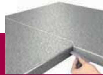
material and the chipboard core. It must be applied with the correct applicator gun to ensure a correctly metered mix of adhesive and hardener.
